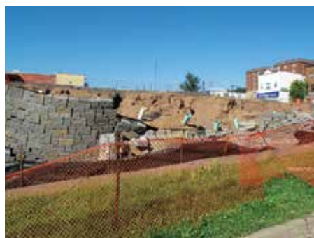
One of our collapsed retaining walls.
