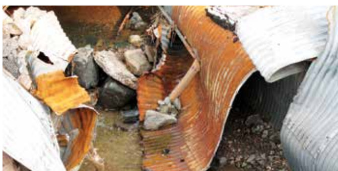
The damaged culvert...
