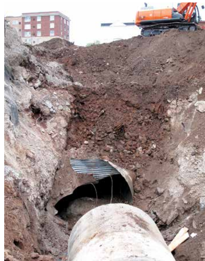
The new culvert begins to be installed...
