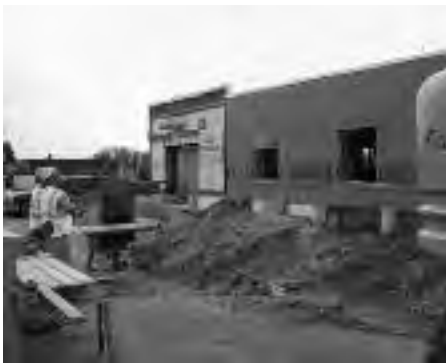
The new facing goes on the front of the store.
